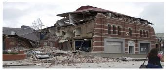
Image of badly damaged low rise buildings during a low to moderate intensity earth quake. This shows the importance of keeping even smaller buildings ductile and seismic resistant.
